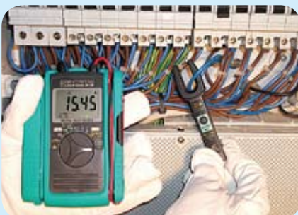
Measuring current in a Switchboard
