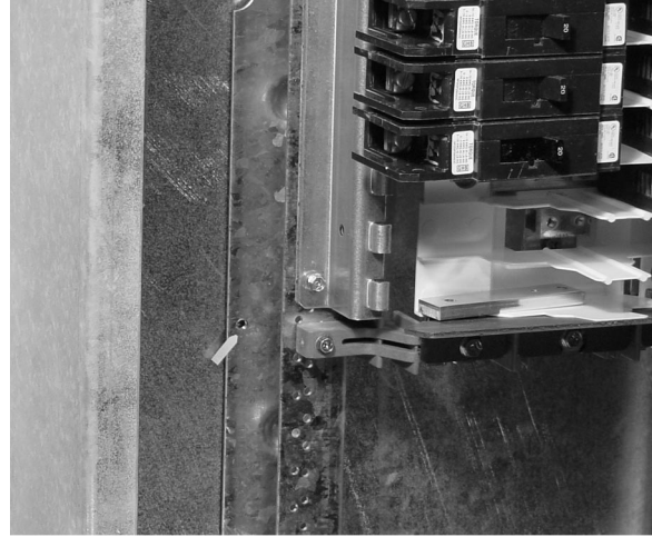
FIGURE 7. LOCATING THE BCB LOWER MOUNTING HOLE
