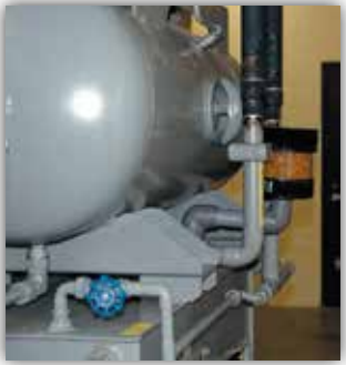
Watchdog Breather installed on a hydraulic reservoir
