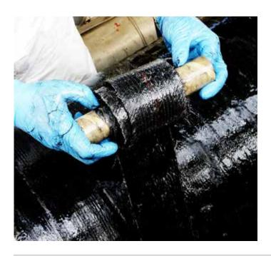
Belzona SuperWrap II is a composite repair solution designed to restore strength to weakened or holed metallic substrates. Developed for applications on pipes and process vessels, it is also suitable for safety critical and pressurised systems, and can be used on bends, tees and other complex geometries.
