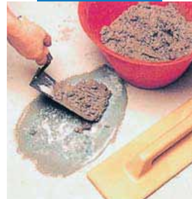
Floor patching: application of mortar
