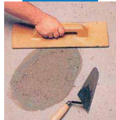
Floor patching: final smoothing
