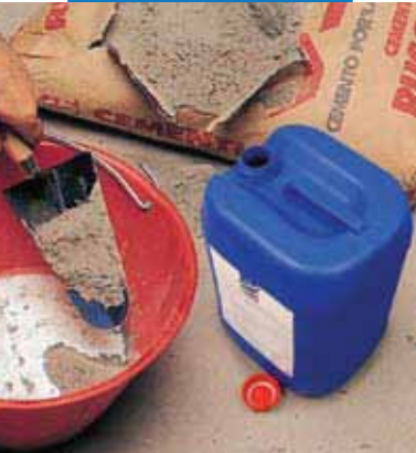
Mixing cement mortar with Planicrete SP for tile fixing
