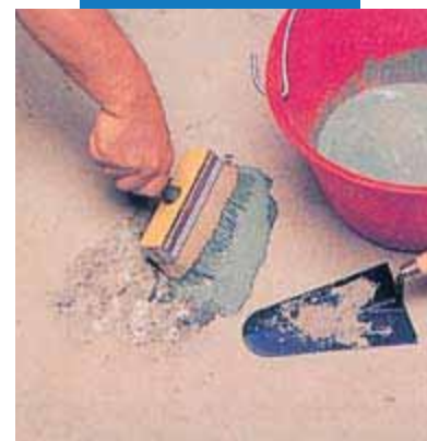
Floor patching: application of slurry
