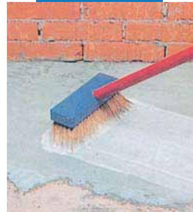
Applying cement slurry modified with Planicrete SP
