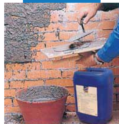
Spatter - dash coat modified with Planicrete SP
