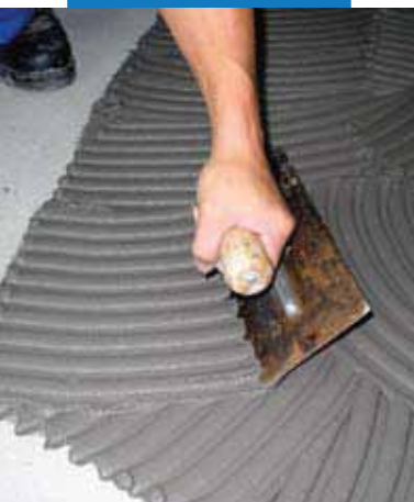
FIXING OF TILES Apply the adhesive onto the prepared substrate using a notched trowel. Do not spread more than 1m 2 at a time.
