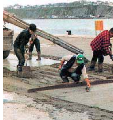
Exterior flooring with concrete admixed with Planicrete SP.
