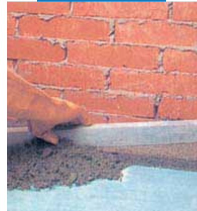
Applying cement screed modified with Planicrete SP
