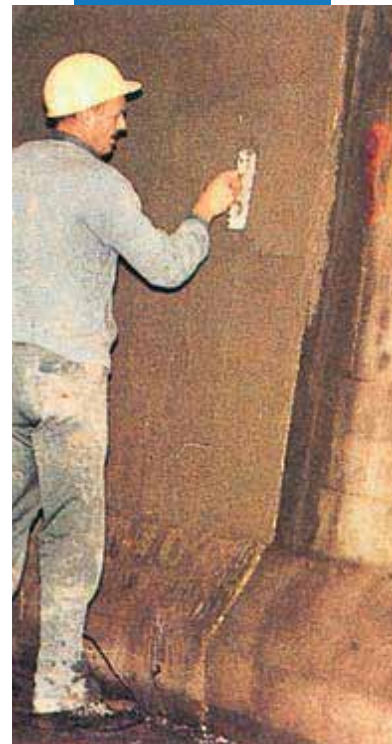
Cement plaster with Planicrete SP.
