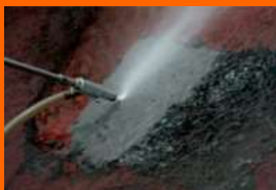
Surface – Sand blasting
