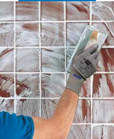
Laying the product with a rubber float
