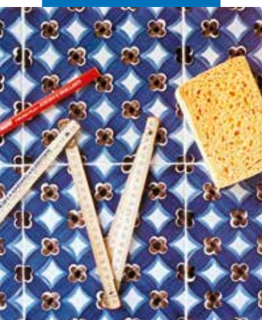
Grouted joints in butt-jointed tiles
