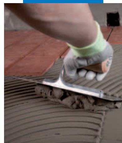
Laying Granirapid on a terrace waterproofed with Mapelastic
