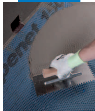
Laying Mapelastic on Mapeket 150
