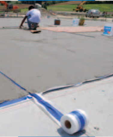
Waterproofing screeds with Mapelastic and Mapeband
