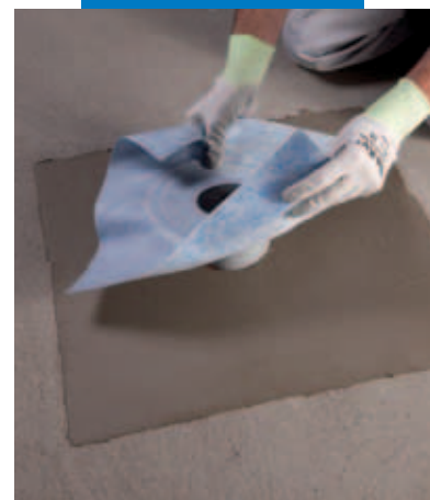
Application of Drain Vertical on Mapelastic
