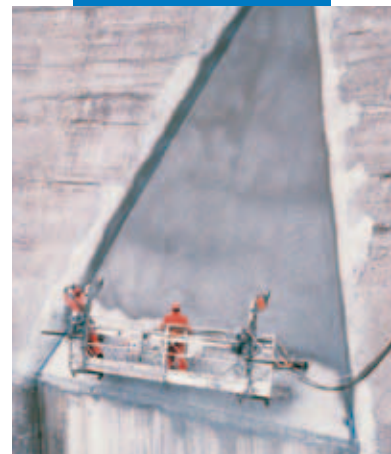
Example of Mapelastic applied on a dam by spraying
