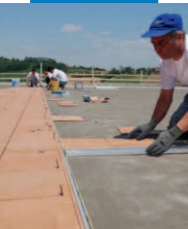
Installing ceramic with Kerabond + Isolastic
