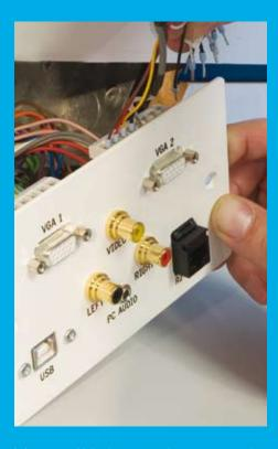
Many AV installations require wall-mounted interconnection plates to allow equipment to be interfaced together as required
