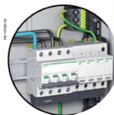
Surge arrester iPRD 4P + iC60N 4P
