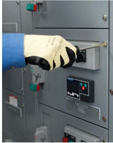
Figure 13: Loosening Captive Fasteners
