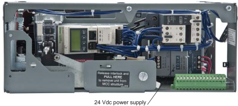
Figure 26: Removing Power Base
