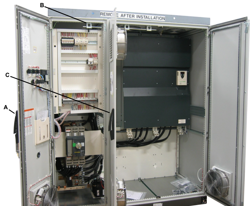
Figure 11: Door Interlock Opening Procedure
