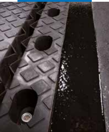
Transition sealed with Mapeflex PU 65 mixed with sand
