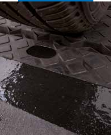
Polymerised Mapeflex PU 65 ready for service
