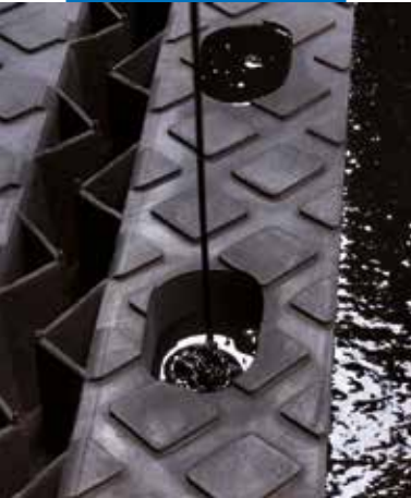
Casting neat Mapeflex PU 65 into the anchorage points
