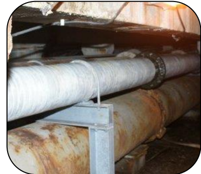
Badly corroded sea water lines encapsulated using 301 Epoxy Resin and hardener and 3 x wraps of Glass Tape
