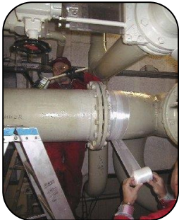
Main fire water lines encapsulated using 301 Epoxy Resin and Hardener and 3 x wraps of Glass Tape
