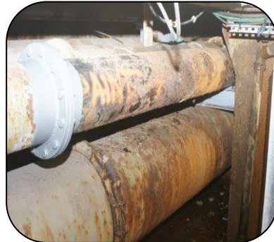
Badly corroded sea water lines encapsulated using 301 Epoxy Resin and hardener and 3 x wraps of Glass Tape
