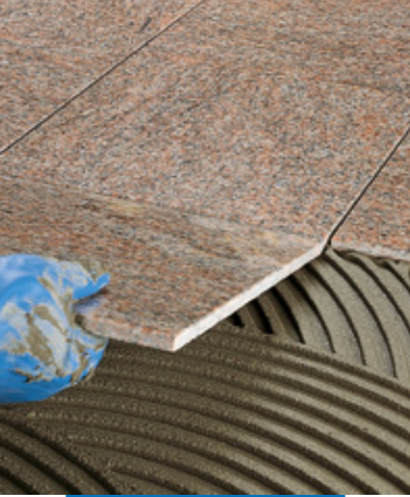
Installation of pre-glossed marble on floors
