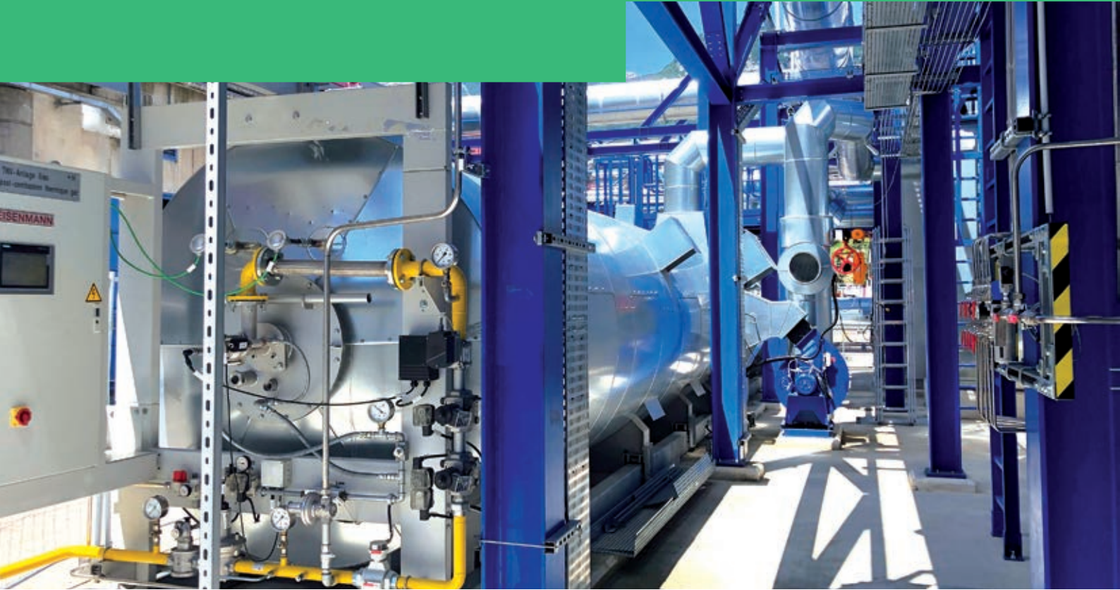
VOC burner, ST Crolles, France
