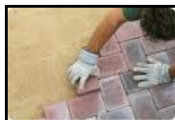
A worker paving the driveway
