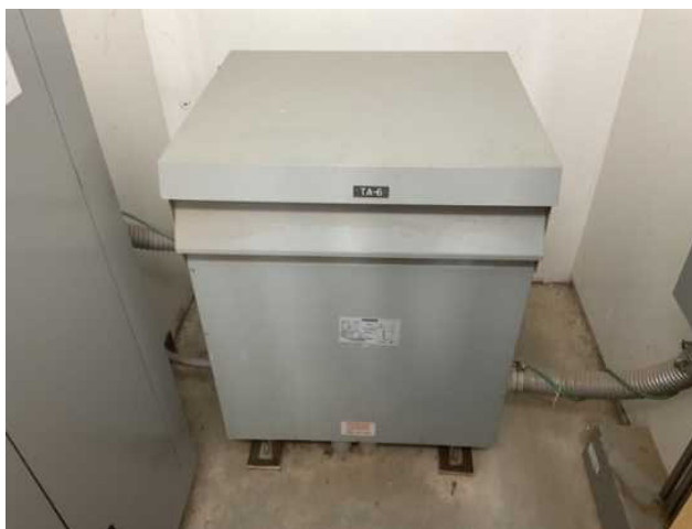
27 - SECONDARY TRANSFORMER
