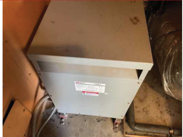
26 - SECONDARY TRANSFORMER
