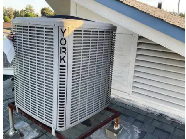
20 - SPLIT SYSTEM CONDENSING UNIT
