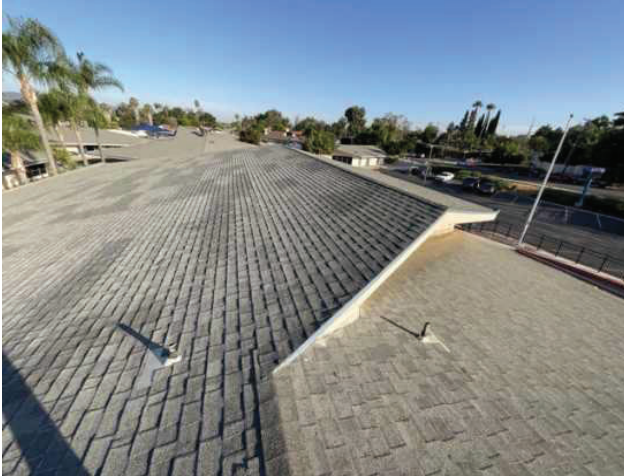
7 - ASPHALT SHINGLE ROOFING
