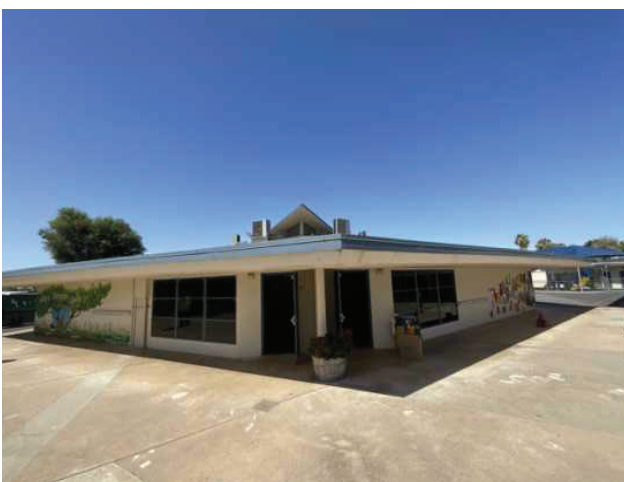
5 - STUCCO WALL WITH LARGE OVERHANGS
