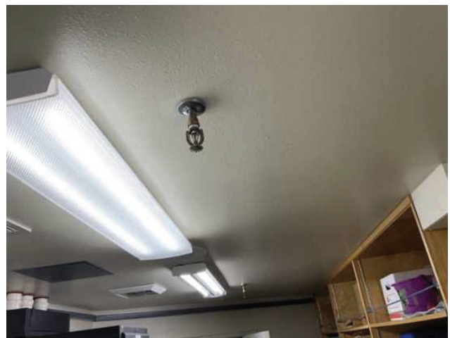
24 - FIRE SUPPRESSION SPRINKLERS
