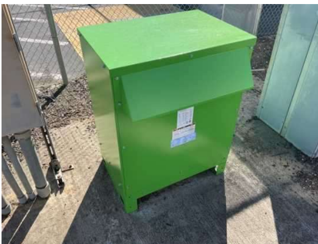
23 - SECONDARY TRANSFORMER
