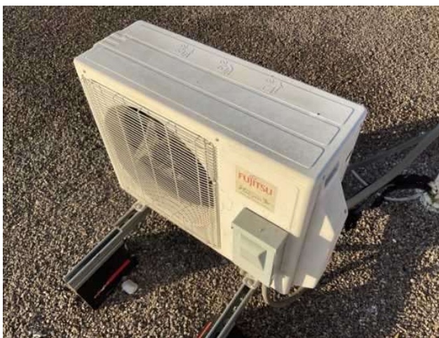
17 - SPLIT SYSTEM DUCTLESS
