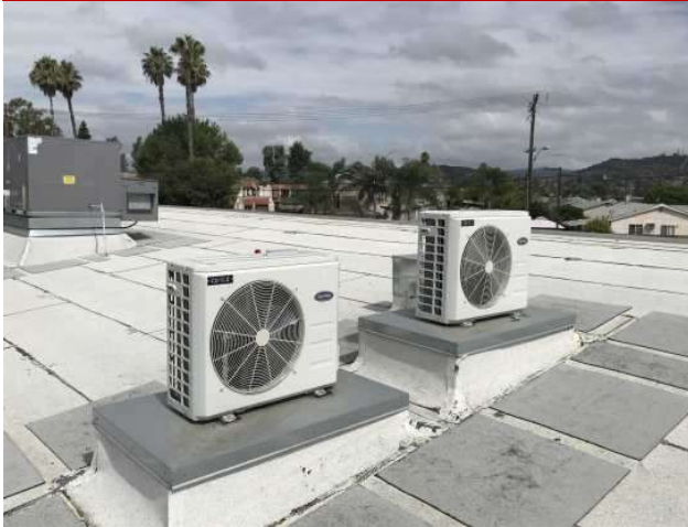
37 - SPLIT SYSTEM DUCTLESS
