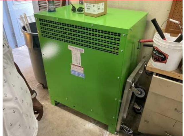
14 - SECONDARY TRANSFORMER
