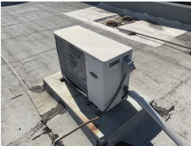
23 - SPLIT SYSTEM DUCTLESS
