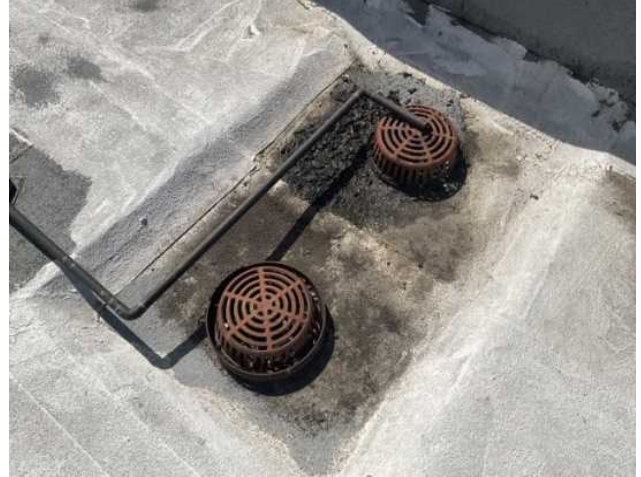
8 - CONDENSATE LINE DRAINAGE ISSUE
