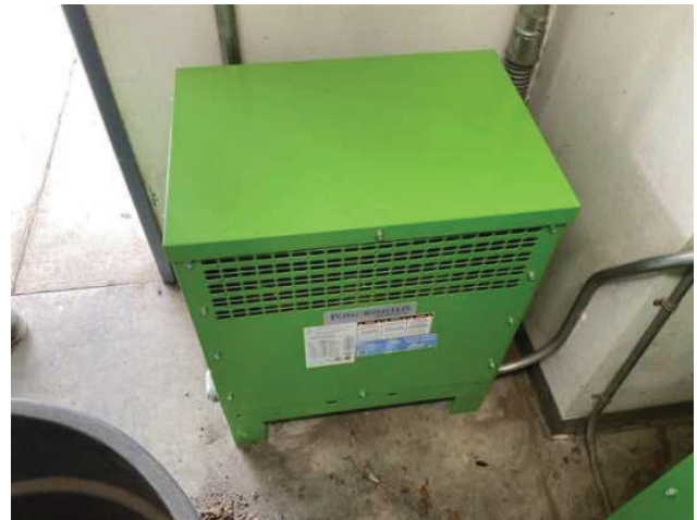
28 - SECONDARY TRANSFORMER
