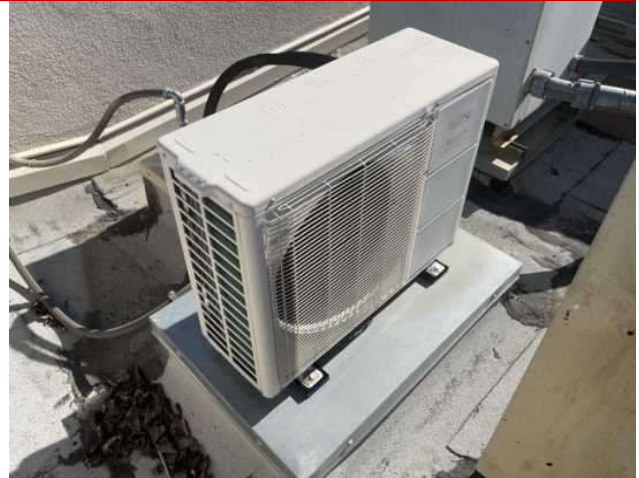
20 - SPLIT SYSTEM DUCTLESS
