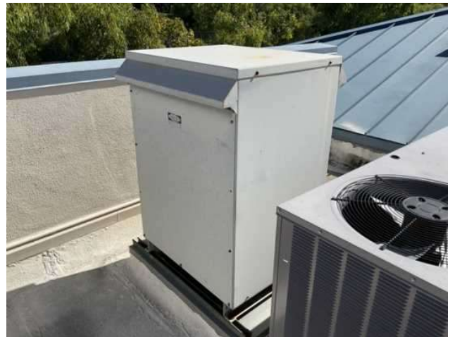
22 - SECONDARY TRANSFORMER
