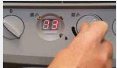
Turn the knob clockwise to increase or anticlockwise to decrease the temperature. Range 25 - 80°C.
