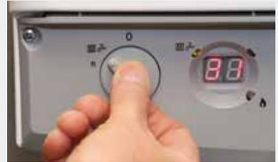
Boiler outlet temperature – In either the central heating or domestic hot water position display will illuminate showing the current boiler temperature in degrees centigrade.
