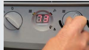
Turn the Central Heating control to set your temperature (this will display for a few seconds). This figure is how hot your radiators are to touch.
