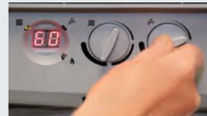
Turn the Domestic Hot Water control to set your maximum water temperature (chosen temperature will display for a few seconds).
