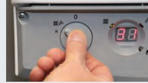
Turn on selector switch (display will show boiler temperature).
