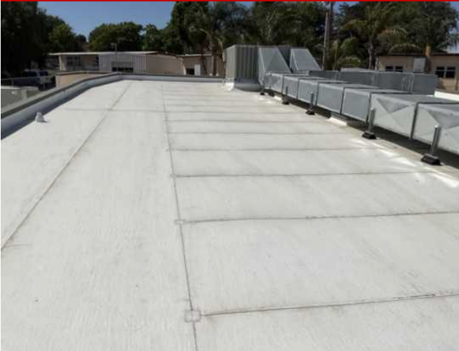
7 - SINGLE-PLY MEMBRANE ROOFING
