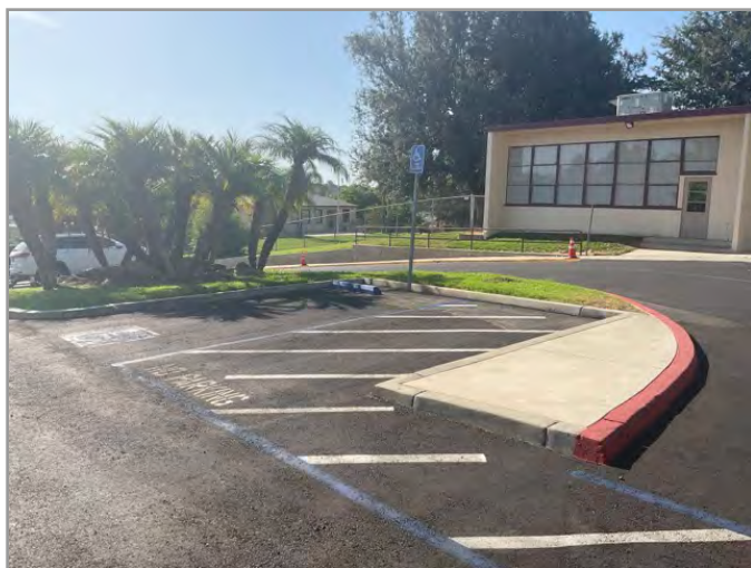
OVERVIEW OF ACCESSIBLE PARKING AREA
