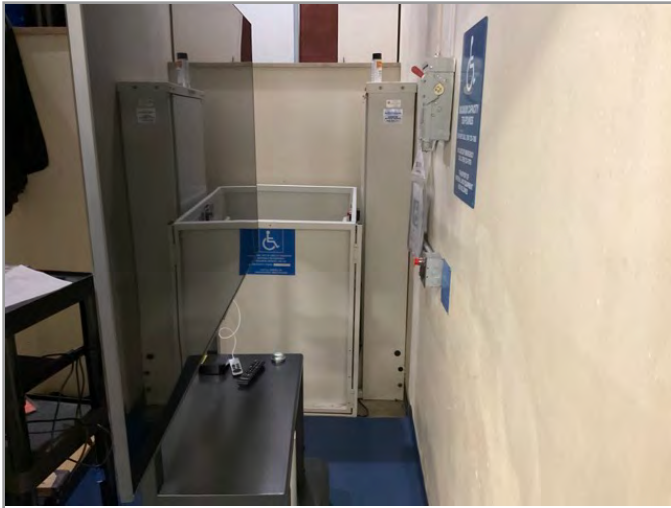
ACCESSIBLE INTERIOR LIFT
