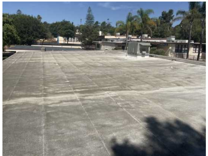
6 - PRIMARY ROOF OVERVIEW
