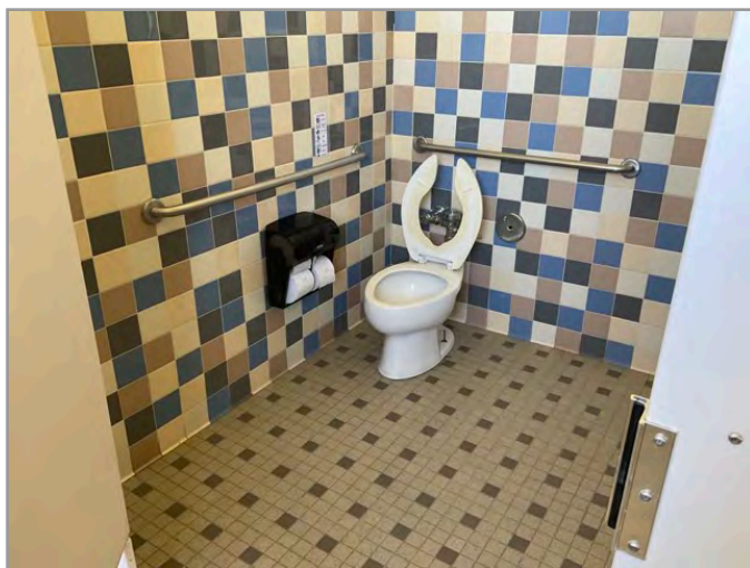
TOILET STALL OVERVIEW
