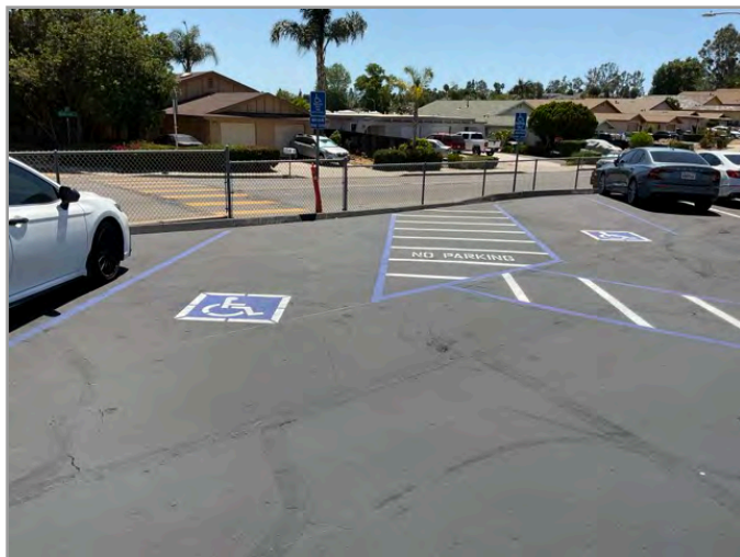
OVERVIEW OF ACCESSIBLE PARKING AREA
