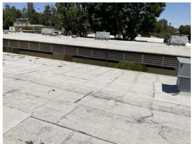
6 - PRIMARY ROOF OVERVIEW
