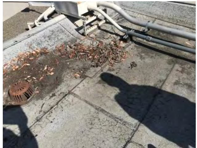
16 - LEAKING ROOF
