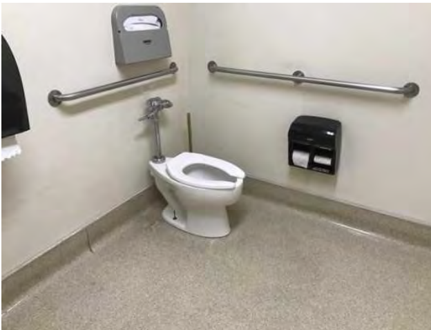
27 - TOILET STALL OVERVIEW
