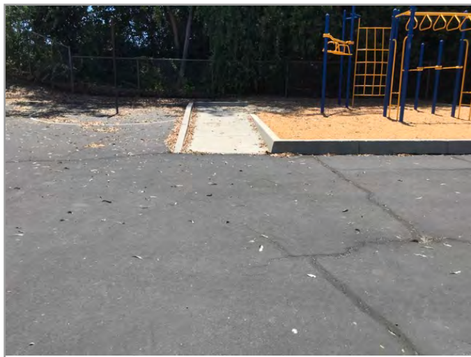
ACCESSIBLE ROUTE TO PLAYGROUND
