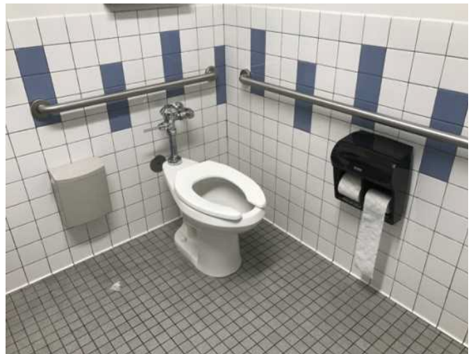
18 - TOILET STALL OVERVIEW
