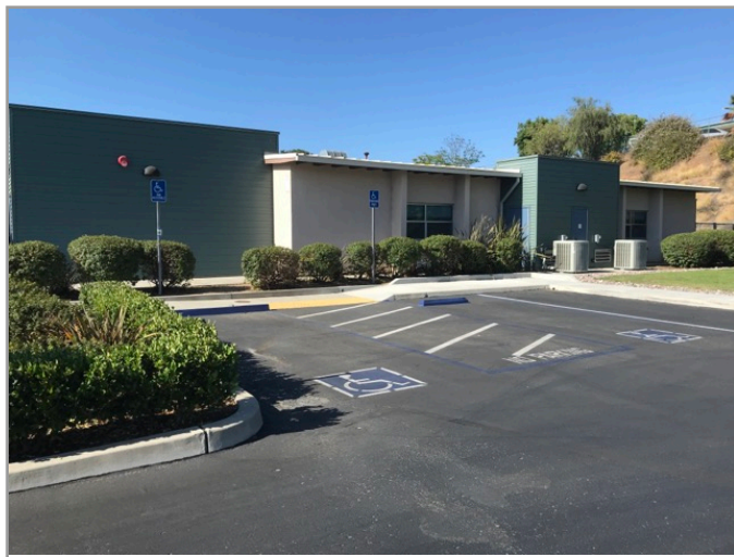
OVERVIEW OF ACCESSIBLE PARKING AREA
