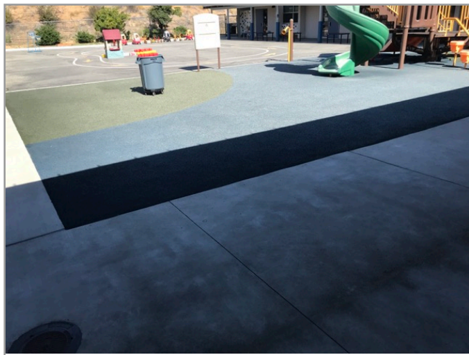
ACCESSIBLE ROUTE TO PLAYGROUND
