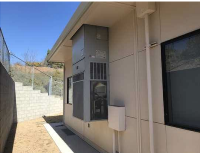
23 - WALL MOUNTED HEAT PUMP
