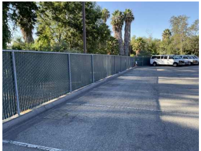
24 - CHAIN LINK FENCE
