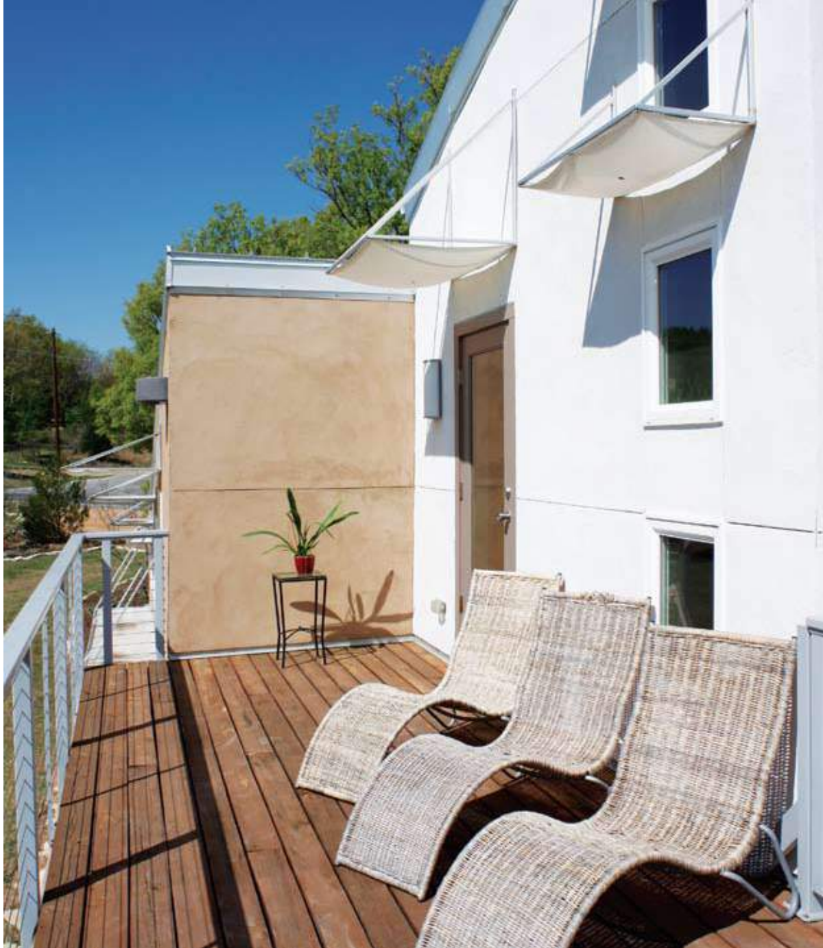
Porches and overhangs provide shade in summer, and canvas awnings retract for natural daylighting.
