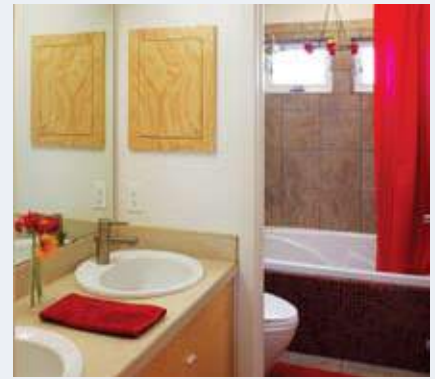
The bathrooms have Delta Brizo low-flow fixtures and dual-flush Toto toilets.
