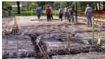
Concrete slab with 51% fly ash replacement
