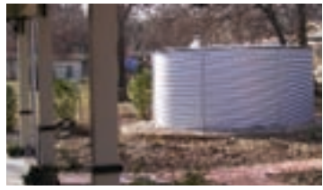
10,000 gallon rainwater collection system for irrigation and whole-house usage
