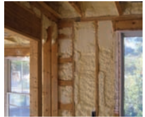
Advanced framing and foam insulation
