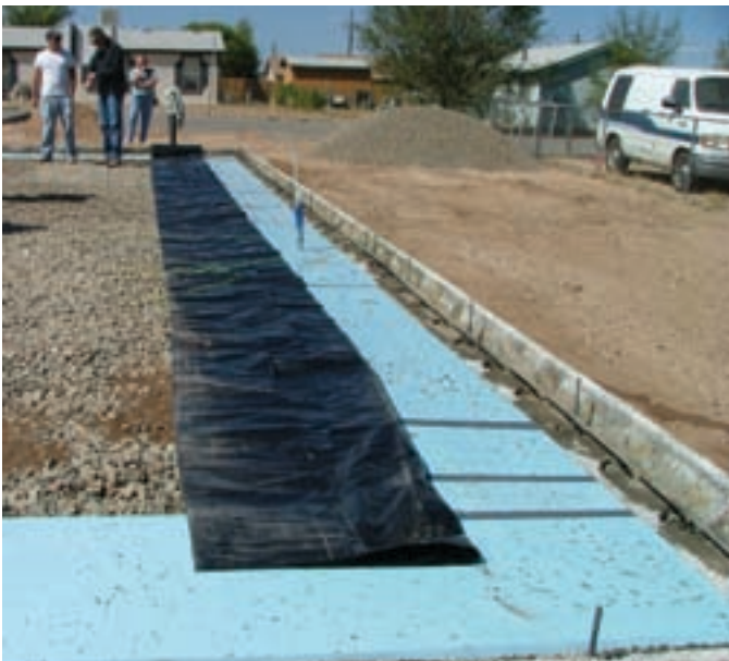
Foundation preparation compaction, gravel, vapor barrier, perimeter insulation
