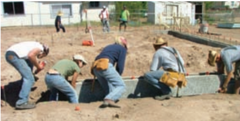
Building site, installation of stemwalls, ICF
