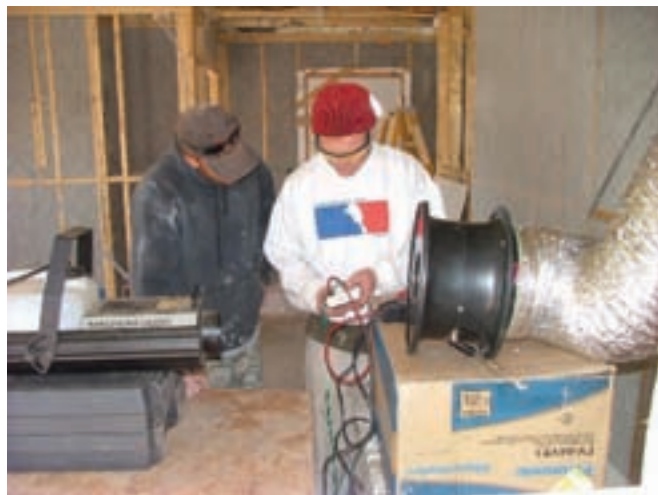
Commissioning testing, duct blaster test
