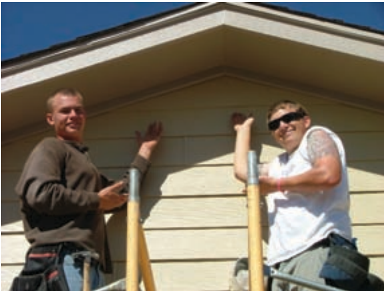
Cementitious siding installation
