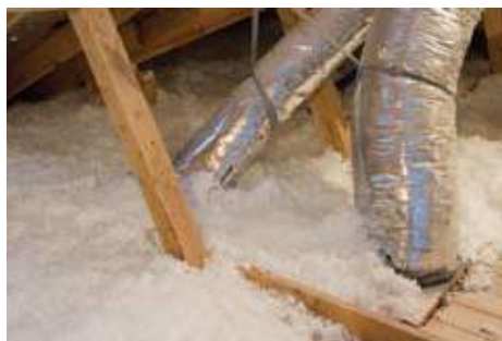
Attic blown-in fiberglass insulation
