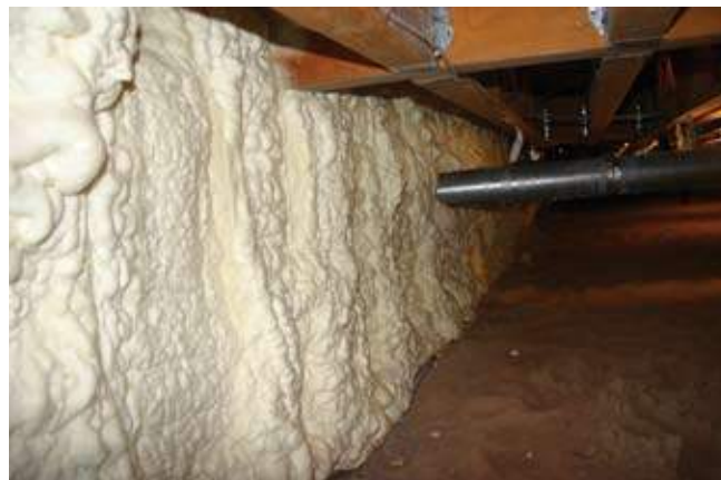
Foam insulation on crawlspace wall
