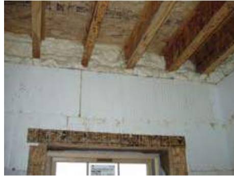
Rim joist sealed and insulated with spray foam
