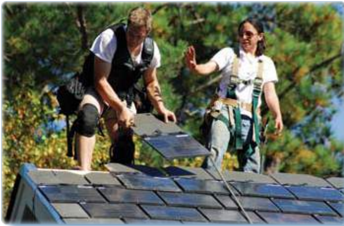
Installation of solar photovoltaic shingles
