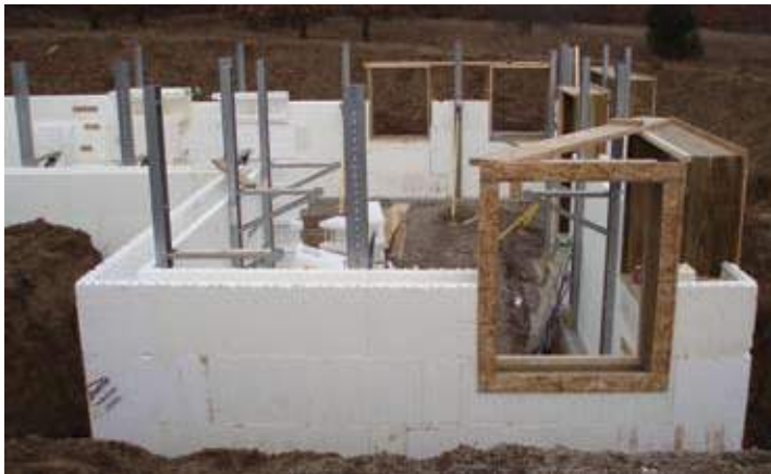
Insulated concrete forms
