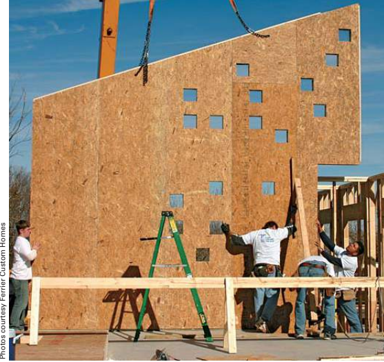
LEFT: A precast structural insulated panel is lowered into place. FAR LEFT: Heather Ferrier in her award-winning home.
