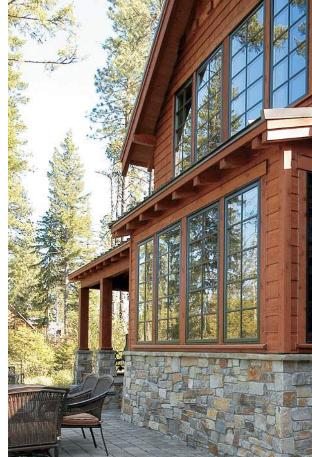
RIGHT, LEFT and BELOW: An indoor air filtration system, geothermal heating and cooling, and an insulated concrete form foundation are some of the components of the lodge-style Built Green home.
