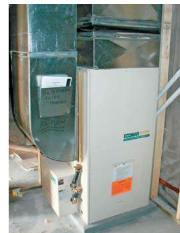
LEFT: An Econar geothermal heat pump system provides heating and cooling for the home.
