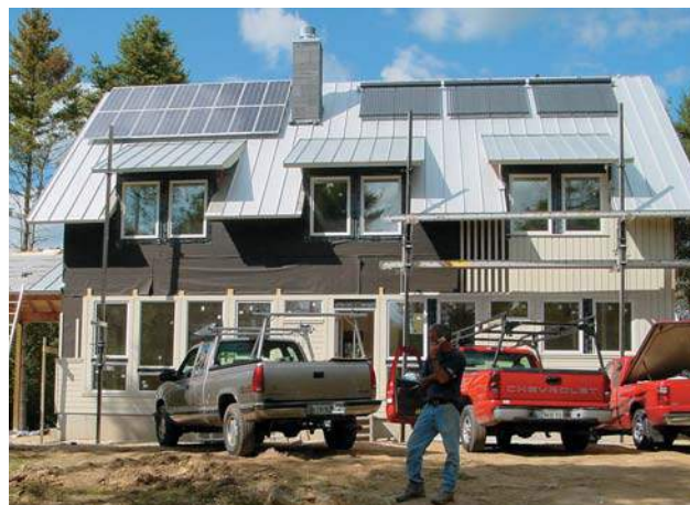
ABOVE and RIGHT: Cranberry Ridge features solar electric and solar water-heating systems on its roof.
