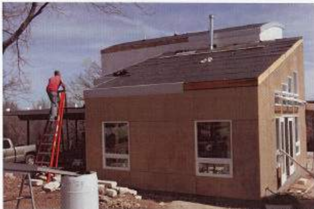
Progress continues on the energy-efficient home being built near Lake Weatherford.
