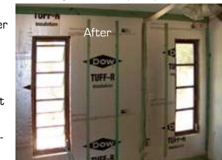
Typical Florida block construction without insulation (above) and a great solution (below).
