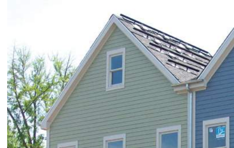
Above: PV support brackets ready for panel installation. Below: Ducts installed completely within the building's well-sealed envelope.
