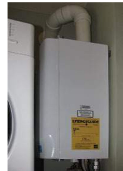
Far left: Solar site surveys—the basis for design and positioning an energy-efficient home. Left: Tankless water heater installed to minimize run lengths to appliances.
