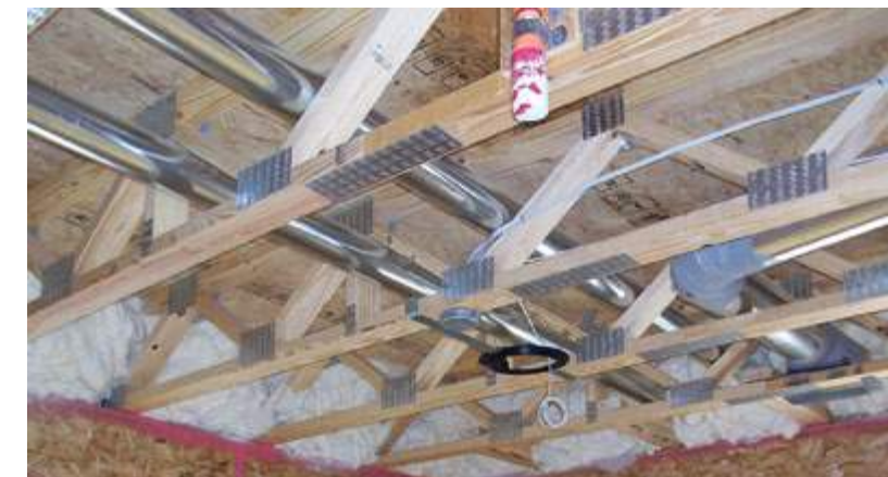
Above: PV support brackets ready for panel installation. Below: Ducts installed completely within the building's well-sealed envelope.
