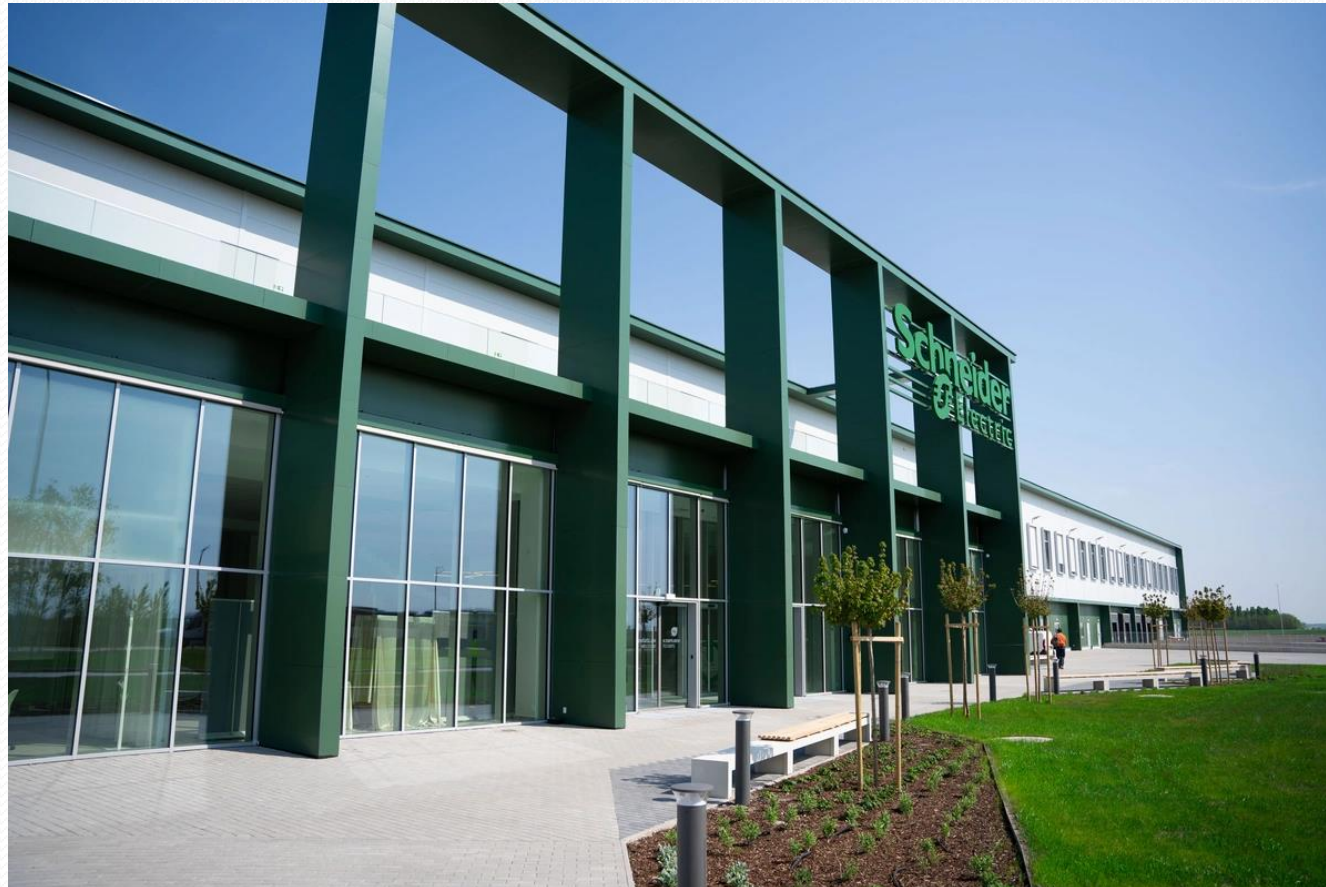
Schneider Electric – Duna Smart Power Systems
