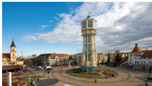
Siófok – City centre rehabilitation
