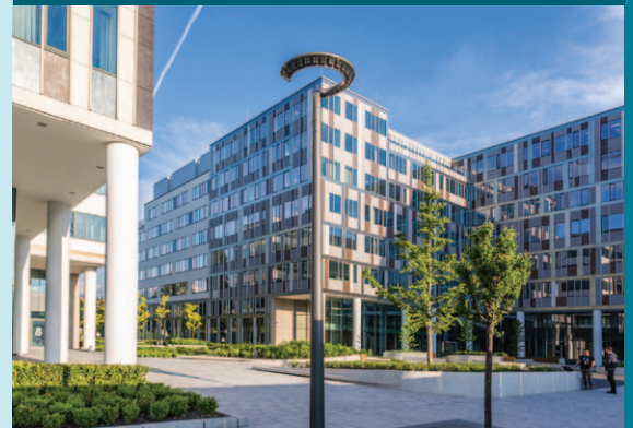
Vaci Greens Buildings A,B,C and D, Budapest
