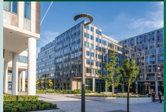
Vaci Greens Buildings A,B,C and D, Budapest
