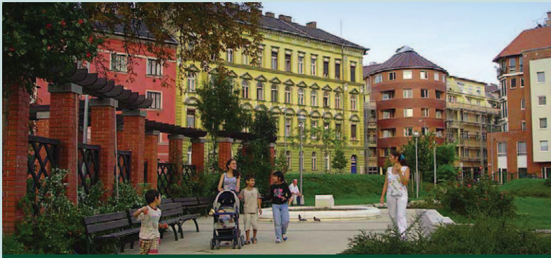
Block rehabilitation in Ferencváros
