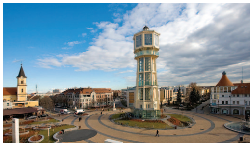
Siófok – City centre rehabilitation
