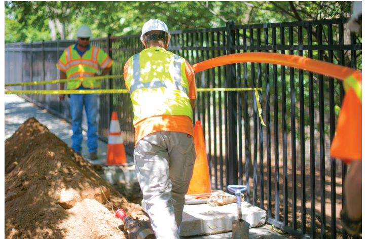
The Fiber team laying conduit in Atlanta, GA
