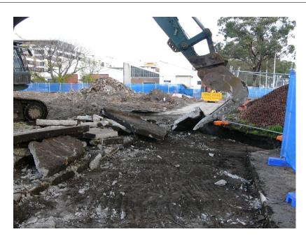
**Figure 6** – Showing method for removal of concrete pavement, by carefully lifting sections and folding over the remaining paved surface.
