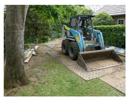
**Figure 4** – Showing typical detail for truck mats.
