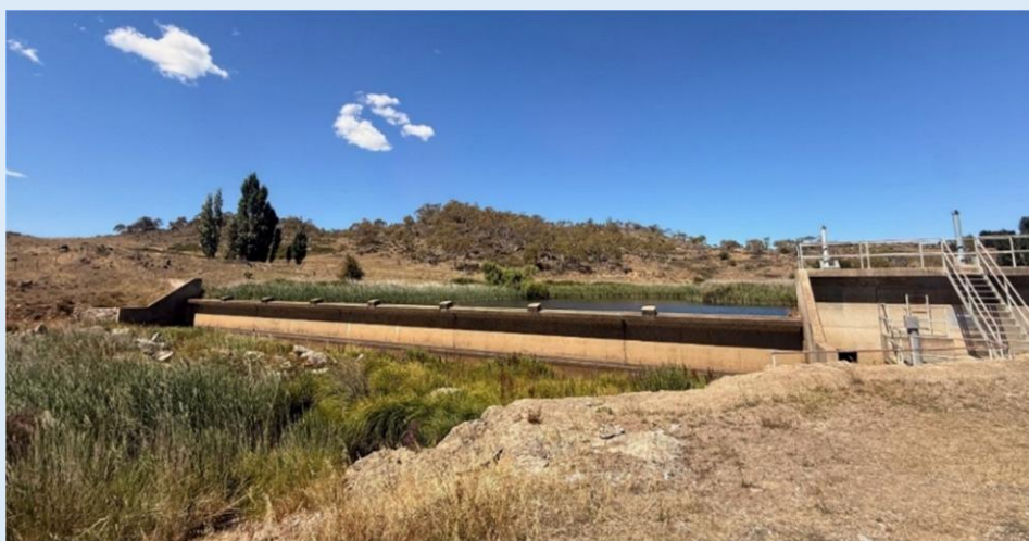
Figure 8: Mowamba Weir, near Dalgety, NSW (February 2026). Source: Australian Government DCCEEW
