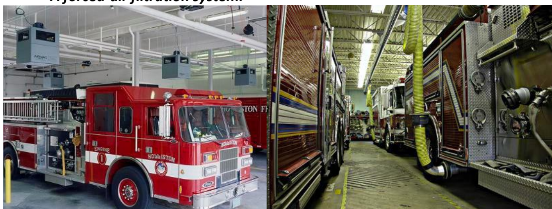
Figure 6.11 — A forced-air filtration system.
