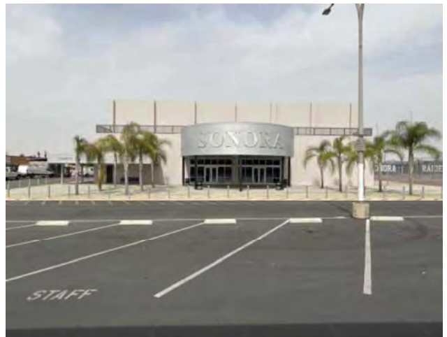
10 - NEW GYMNASIUM BUILDING
