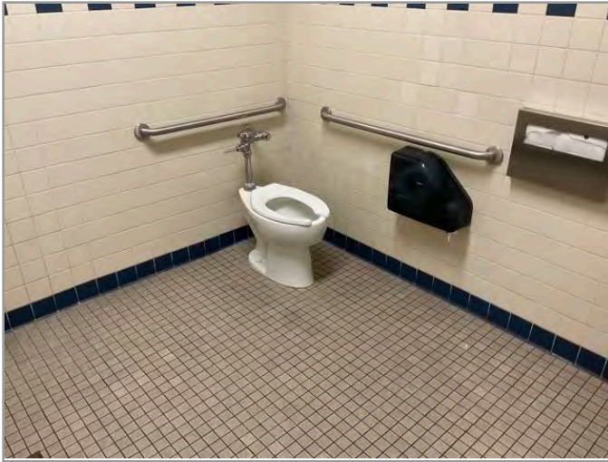
TOILET STALL OVERVIEW
