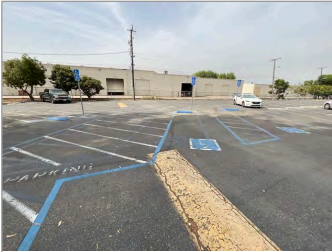
OVERVIEW OF ACCESSIBLE PARKING AREA
