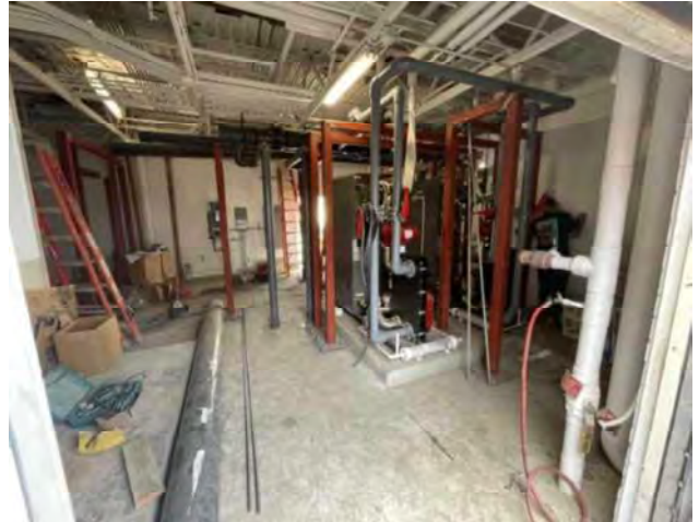
20 - POOL EQUIPMENT ROOM (UNDER CONSTRUCTION)
