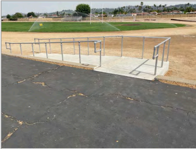
ACCESSIBLE ROUTE TO PLAYGROUND
