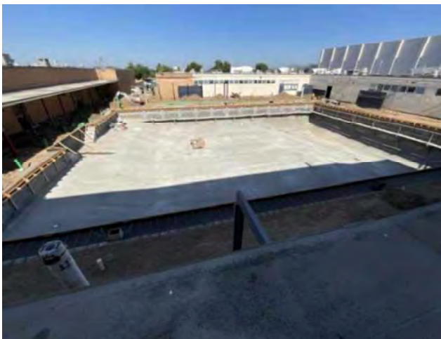
35 - POOL (UNDER CONSTRUCTION)
