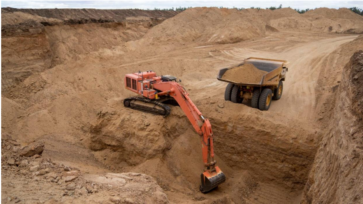
Figure 4. Heavy equipment is used to extract the weathered basalt layers. Over time, they have turned into reddish sands and clays, which can be easily dug out with an excavator without the use of explosives. In some cases, river systems have washed away the sands and only left behind the heavy minerals, including sapphires. Photo by V. Pardieu/GIA.
