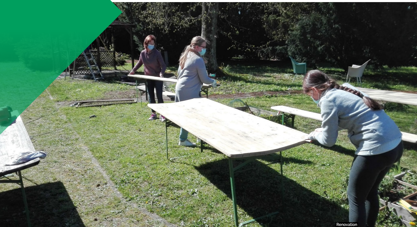
Renovation of a pergola
