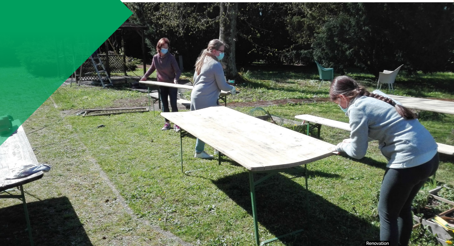
Renovation of a pergola
